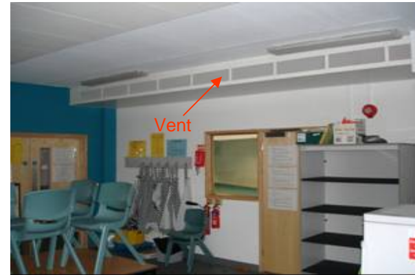
Cross Ventilation from a classroom
