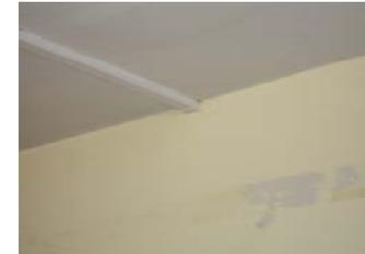
Cable and other holes are required to be made good
