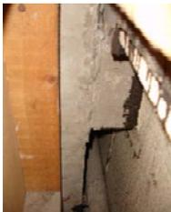
Gap at junction between walls and façade required to be infilled
