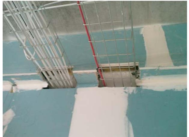
The details below are required to be fully sealed with patress panels, with an equal mass to that of the partitions. All holes are to be sealed with mineral wool and non hardening mastic, including the opening to the trunking.
