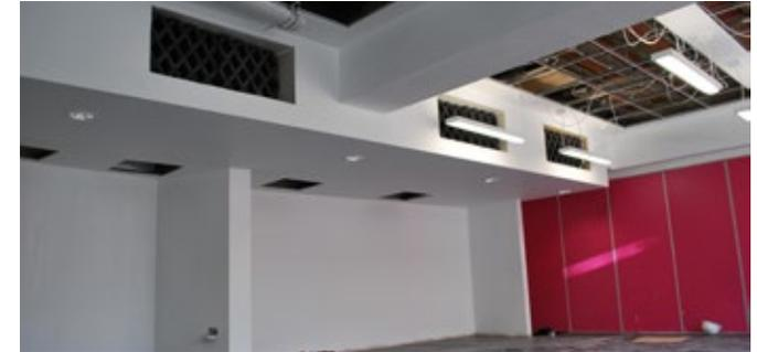
Cowllins Construction completed the installation of the NAT Vent attenuator by means of adding grill to the above units (not pictured). As smoke vents, louvres were fitted at the tapered end of the ducts.
