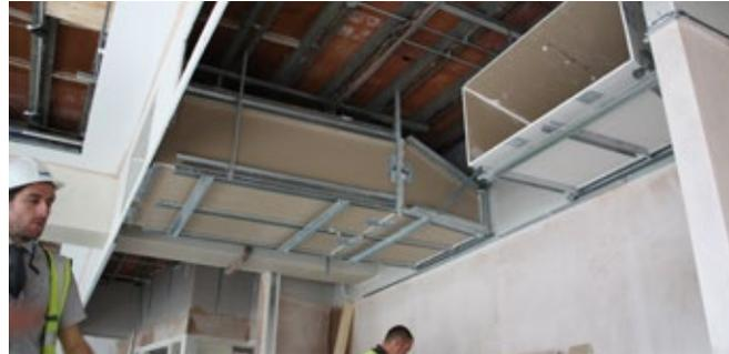
For the Attenuators to be efficient, they have to be acoustically enclosed so the noise cannot bypass the attenuators. Our solution here was to install the attenuators into a pre-constructed duct; forming an NVA Box.
