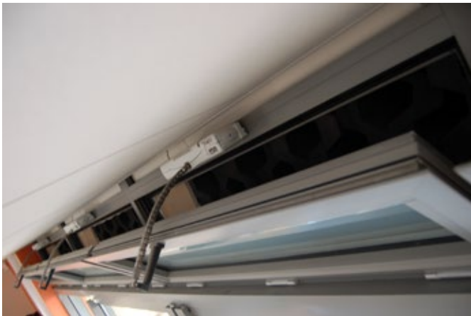
Following the construction of a plasterboard bulkhead, the NVA foam is slid into place in layers to form the honeycomb arrangement
